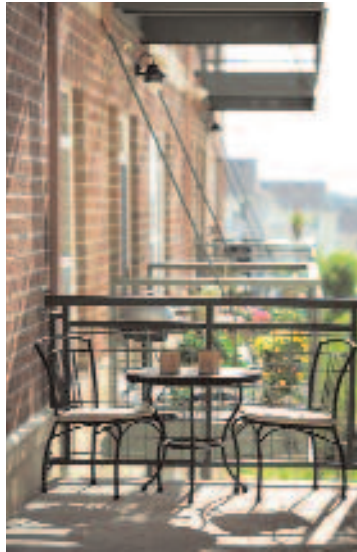
Lincoln Square Lofts' attractive detailing with an industrial edge reinforces the notion of loft living.
